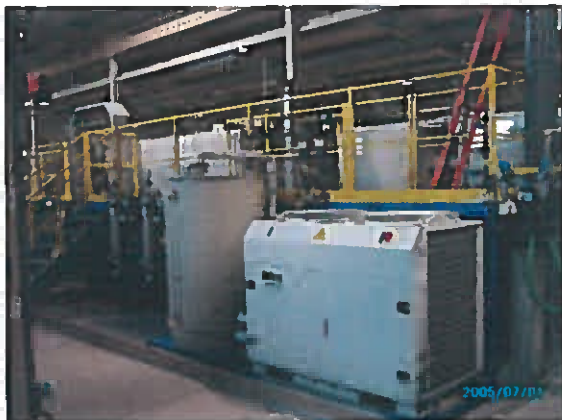
Parts of EC plant (chiller)
